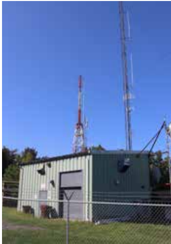
WRGB's former analog transmitter site atop the Helderberg Mountains in New Scotland
