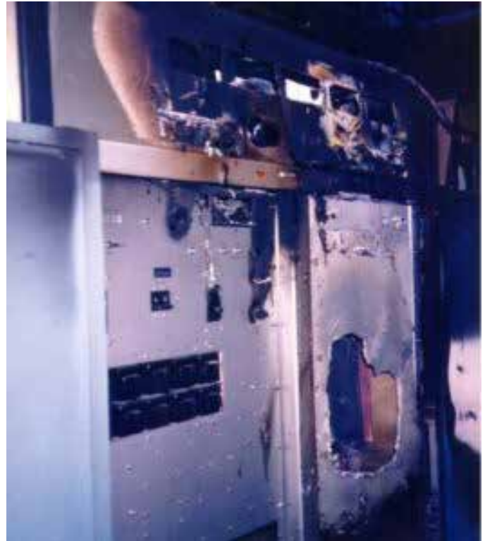
Here is what one of those transmitters looks like after a fire -- if one is lucky enough to extinguish it before it destroys the whole site.
